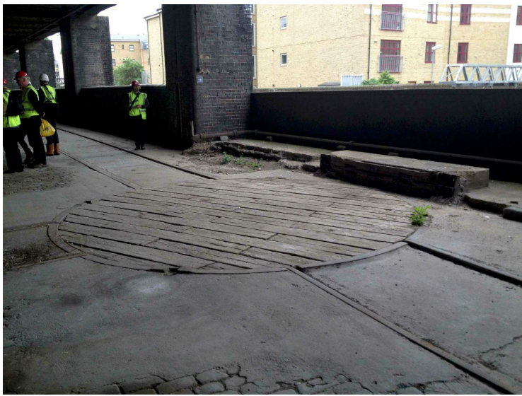
EXAMPLES OF EXISTING GOODSYARD FEATURES (eg. cobbles, railtracks, turning tables etc) THAT WILL BE RECOVERED FOR RE-USE IN NEW DEVELOPMENT - See Spacehub Landscaping Proposals.
